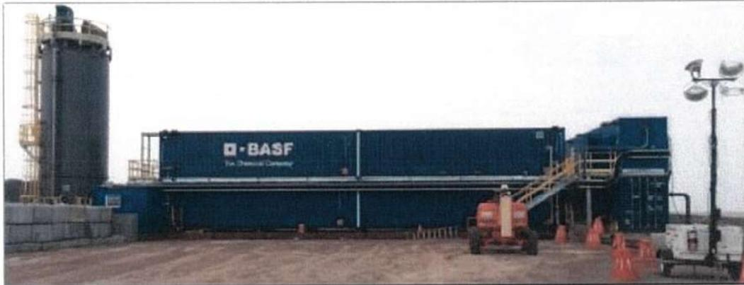
Above: Large CPS (Continuous Polymer System) Plant – 1400kg/hr Polymer powder capacity at 256m<sup>3</sup>/hr
